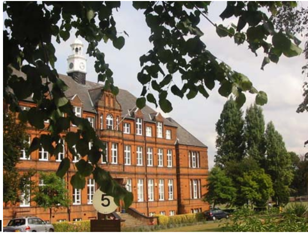
Alleyn's School, Townley Road, An impressive late 19 th century red brick educational establishment, set in and amongst large, open grounds. The original clock tower is mirrored by a modern clock tower on a new pavilion to the south. It is unlisted but is a key building as a focus to views across the sports grounds and as a counterpoint to the spire of St. Barnabas' Church on the ridge to the south.
